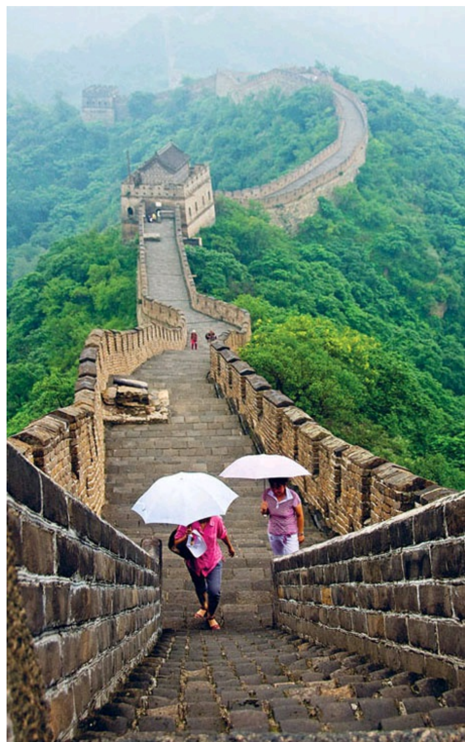
Part of the wall at Mutianyu, northeast of Beijing TIM MAKINS / GETTY IMAGES ©
