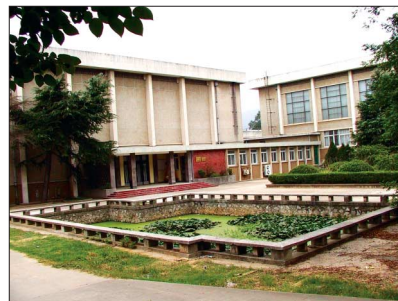
Exterior of the badminton hall
