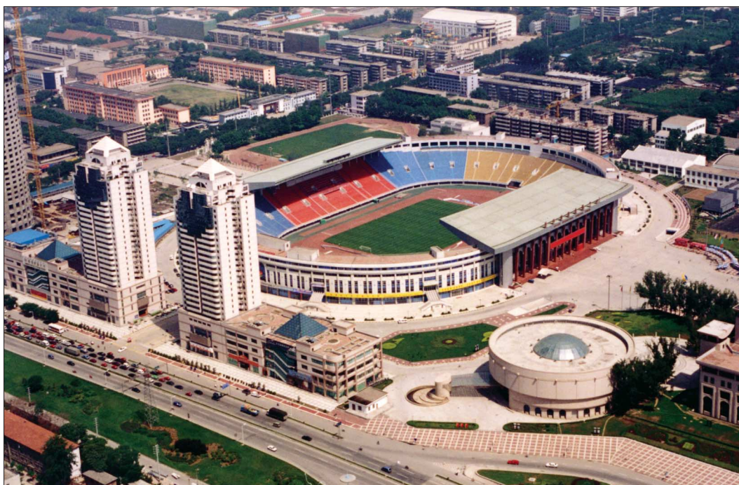
Shaanxi Provincial Stadium
