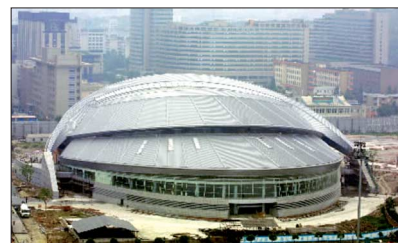
Zhejiang Huanglong Sports Center Stadium
