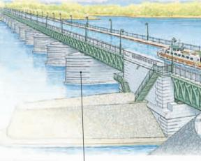
The 15 granite piers supporting the structure were bedded using early compressed-air techniques.
