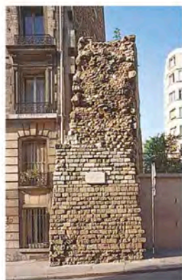
Part of the medieval city wall near Place de la Contrescarpe
