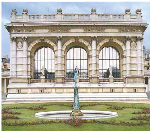
Garden and rear façade of the Palais Galliera
