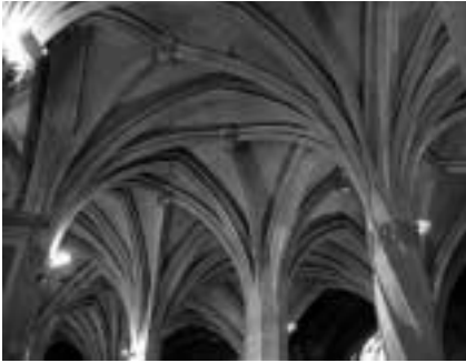
▲ FLAMBOYANT VAULT AT ST-SEVERIN
