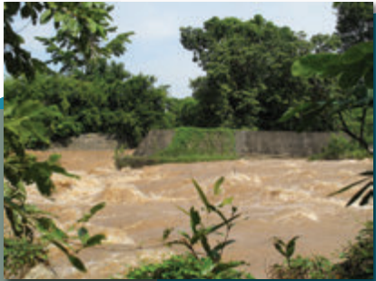
Teak diversion wall seen from Don Pa Soy
