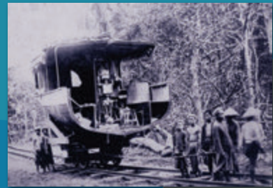
The railway bypassed the rapids to transport disassembled steamers from Hang Khone to Ban Khone.
