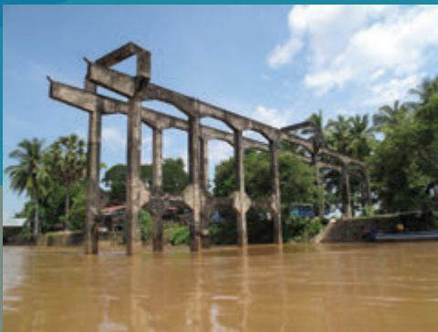
Ban Don Det gantry's reinforced concrete structure and pier
