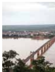
The Japanese bridge
